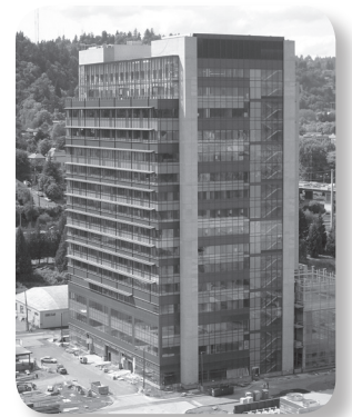
Oregon Health & Science University Center for Health & Healing, Portland LEED Platinum (pending) Total cost premium - 1%. Photo: Interface Engineering, Inc.
