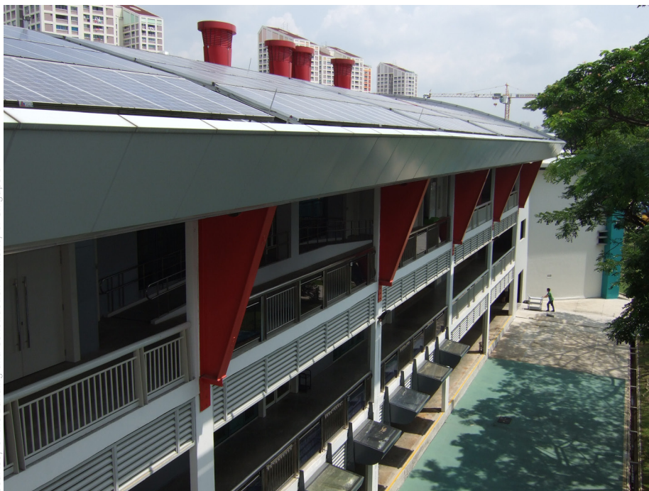
About 1,540 square meters of roof- and façade-mounted photovoltaic panels are connected to grid power supply and generate about 207,000 kWh a year.
