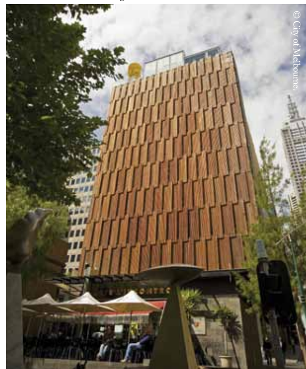
Figure 1: A 6-Star Green Star-rated building, Council House 2 in Melbourne, Australia, pioneered an urban innovation, 'sewer mining' of blackwater for treatment and reuse in buildings.
