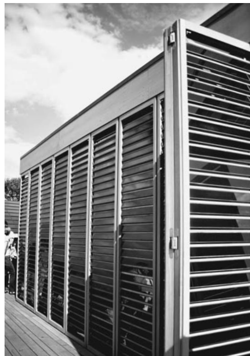
FIGURE 1.3 The German student entry won the 2007 Solar Decathlon, producing more energy than it consumed using building-integrated photovoltaic systems. (Kaye Evans-Lutterodt/ Solar Decathlon )
