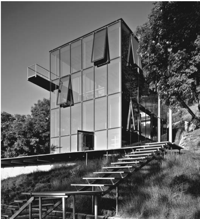
FIGURE 1.4 Werner Sobek's all-glass house in Stuttgart uses trans-seasonal thermal storage to provide heating in winter, along with solar photovoltaic and thermal panels.
