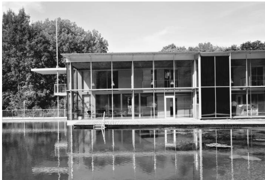
FIGURE 1.5 Georg Reinberg's B!otop office in Austria uses a full range of integrated design strategies to create a low-energy building.
