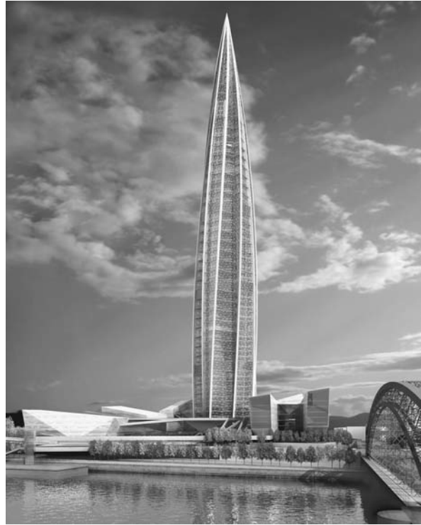
FIGURE 9.7 Slated to be Europe's tallest building, RMJM's Okhta Tower in St. Petersburg, Russia deals with a very cold climate in imaginative ways. (RMJM)
