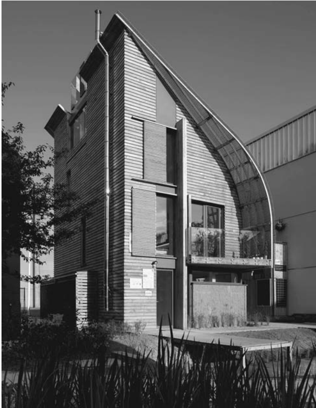
FIGURE 9.5 With a strong commitment to zero-carbon housing, the United Kingdom is pioneering stylish sustainable buildings such as this home, designed by Sheppard Robson. (Sheppard Robson)
