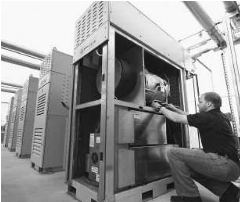
Capstone Turbine Corporation
