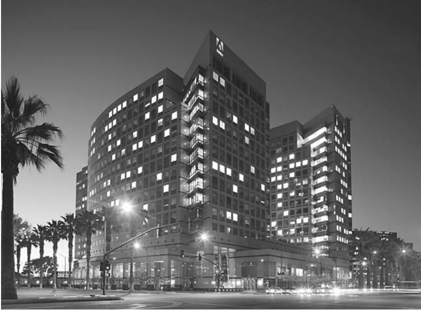
Figure 14.1. Adobe Systems demonstrated its commitment to environmental stewardship with three LEED-EB Platinum-certified buildings on their San Jose campus. Photo by William A. Porter, courtesy of A&R Edelman.
