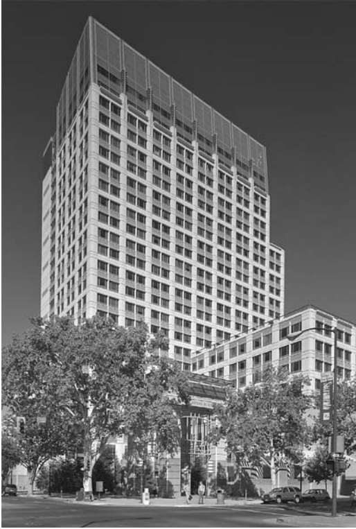
Figure 14.2. The LEED-EB Platinum-certified California Environmental Protection Agency building uses 34 percent less energy than a comparable building. John Swain Photography, courtesy of Thomas Properties Group, Inc.
